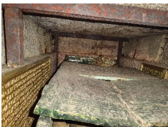
View into the tomb looking west, showing the coffin made of glazed ceramic tiles, the inscribed tablets on the north and south walls, and the funerary crown that extends beyond the slabs comprising the lid © Dombauhütte zu St. Stephan
